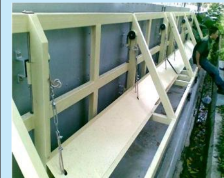
Flood Protection Gate Installation. Protect from flood of sea water tide - Jakarta
