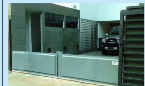
Flood Protection Gate Installation. Protect from flood of sea water tide - Jakarta
