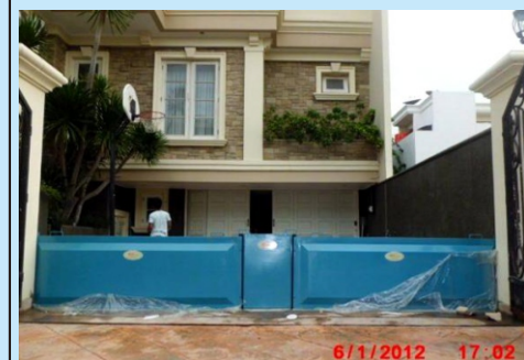
Flood Protection Gate Installation Pantai Mutiara Residential-Jakarta
