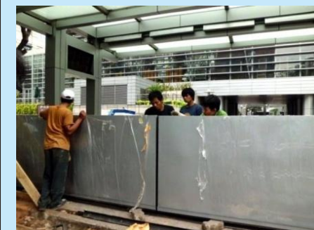
Flood Protection Gate Installation Pantai Mutiara Residential-Jakarta
